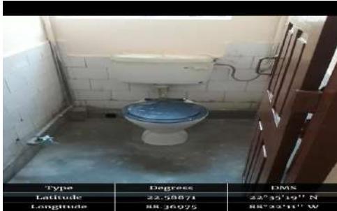
SINGLE TOILET BLOCK IN LADIES COMMON ROOM
